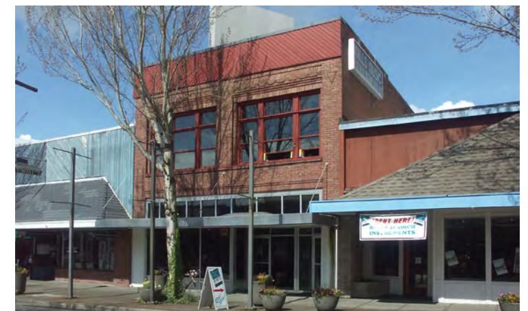
FIG. 1.12 HIDDEN HISTORIC ASSETS - NOW While some details were removed for seismic reasons, many historic Main Street facades have been remodeled with unsympathetic claddings and awnings.
