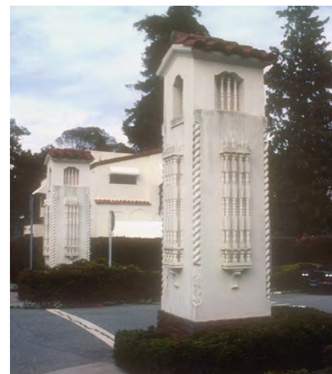
FIG. 2.43 EXAMPLE OF TRADITIONAL NEIGHBORHOOD GATEWAY WITH ARCHITECTURAL STYLE CHARACTER RESEMBLING NEARBY HOMES
