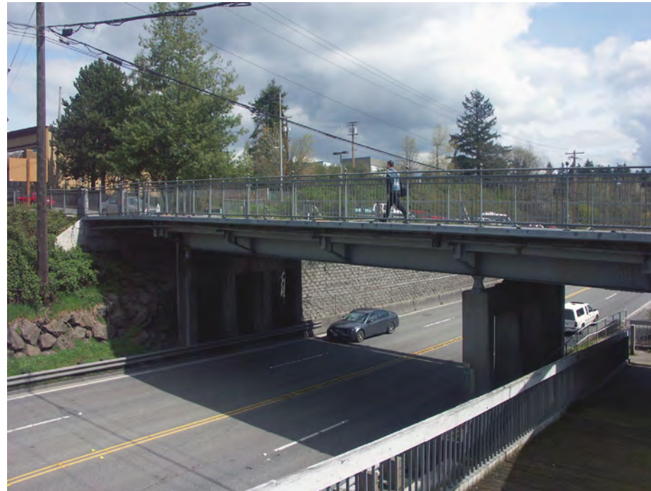
FIG. 2.35 VIEW TOWARDS NORTH-EAST OF RECONSTRUCTED 102 ND AVENUE NE BRIDGE AT SR 522.
