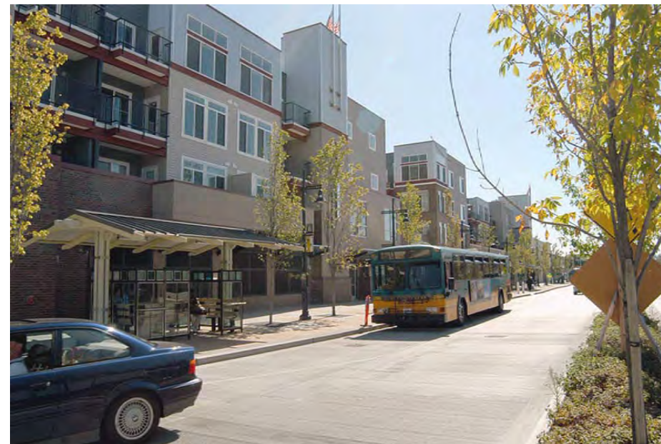
FIG. 2.57 EXAMPLE OF TRANSIT-ORIENTED STREET - BURNETT AVENUE IN RENTON, WA (Photo provided by Perteet Inc.)
