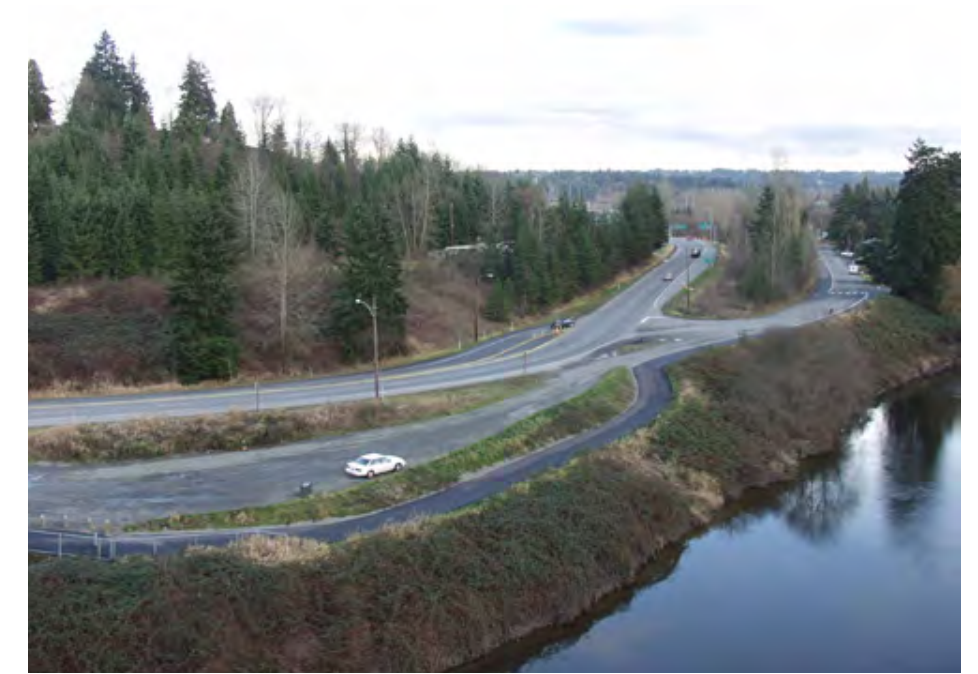
FIG. 2.32 PHOTO OF EXISTING SITE OF FUTURE UWB/CCC SOUTH CAMPUS ACCESS AT SR 522
