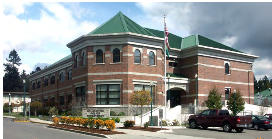
FIG. 1.31 BOTHELL POLICE DEPARTMENT BUILDING
