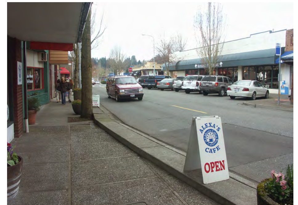
FIG. 2.21 EXISTING PROTRUDING SIX INCH HIGH CURB ON SOUTH SIDE OF MAIN STREET
